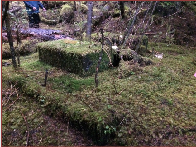
Concrete foundation for power plant shelter
