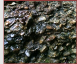
Close-up of concrete poured with local aggregate
