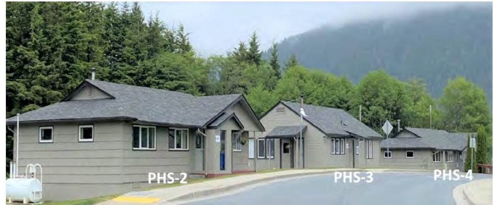
PHS Building on Tongass Drive, 2019
