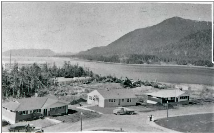
PHS Building on Tongass Drive, ca. 1950s
