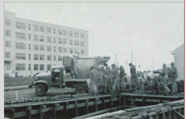
Pouring foundation for PHS building (BIA - Mt. Edgecumbe Yearbook, TAHETA 1958)
